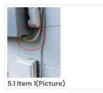
(2) DANGER - Is the lightest way to say whoever dropped this screw into the electrical panel had one lucky day. I talk a lot to Homeowner about screwing into panels and can't stress enough about the use of pointed screws going into Electrical Panels.
